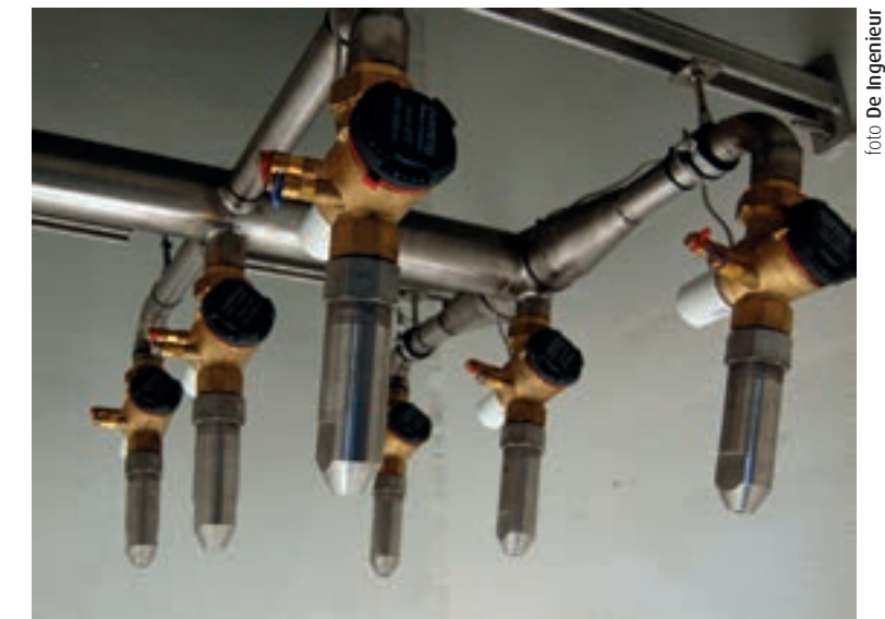
The climate cascade's sprinklers help with ventilation at the Breeze Hotel. The droplets from these sprinklers trigger the airflow.
